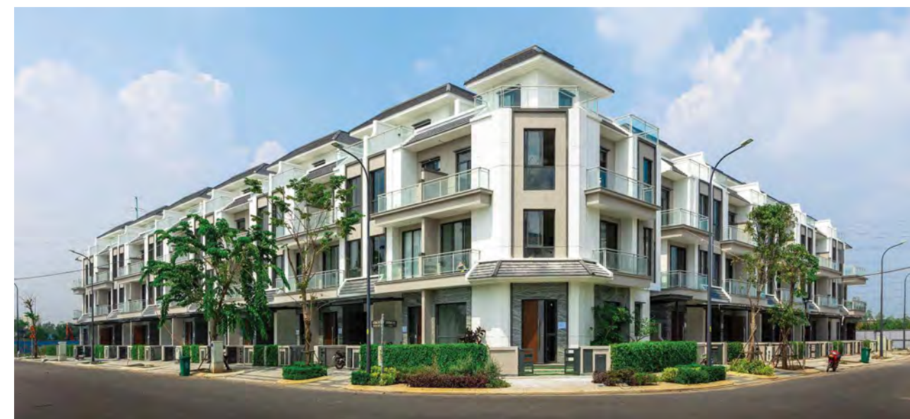
Construction site of Residence area in Binh Trung Dong 1 and Binh Trung Dong 2
